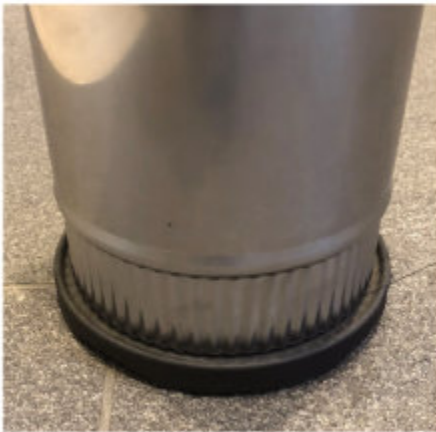
Flue seated correctly.
