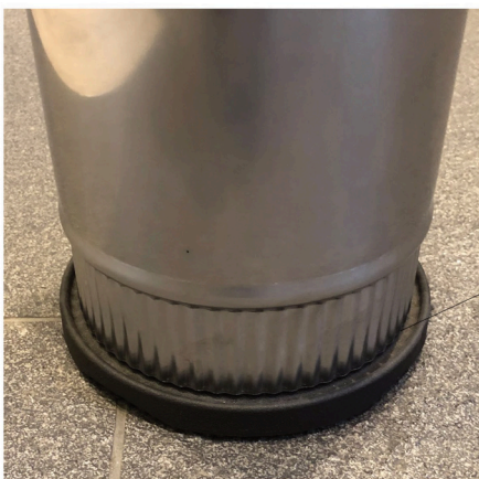
Flue seated correctly.
